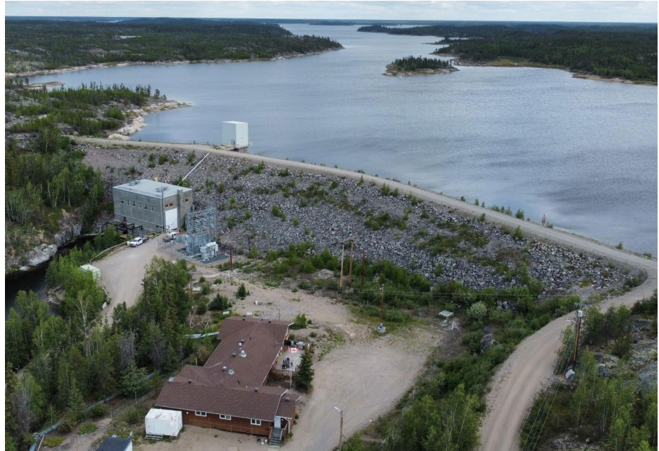
Snare Rapids Main Dam and Powerhouse
