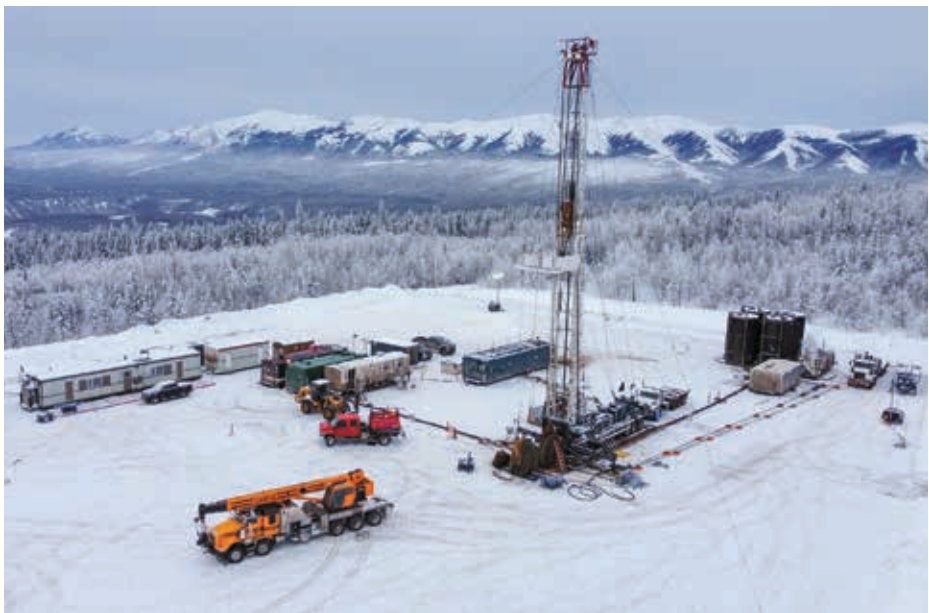
Well abandonment operation near Fort Liard, February 2026.
