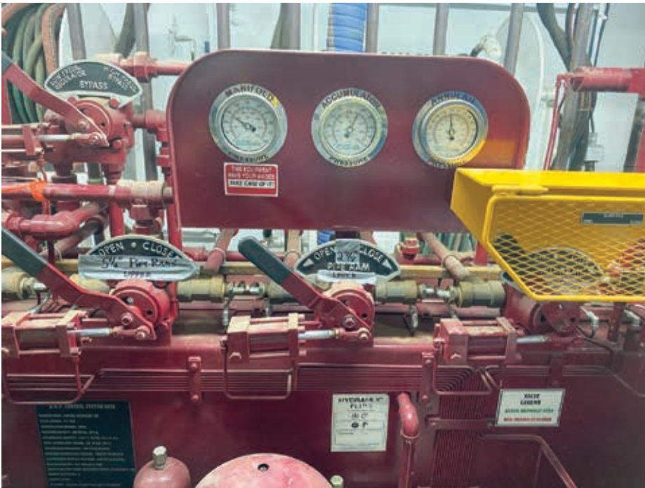
Accumulator near Fort Liard, February 2026. (Credit: OROGO)
