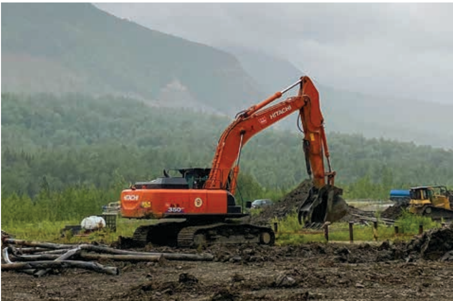
Site abandonment operation near Fort Liard, July 2025. (Credit: OROGO)
